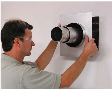
4. Mount the backing plate from the inside of the structure and fasten it with appropriate hardware.
