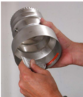
13. Apply a bead of sealant to the inside of the adapter.
