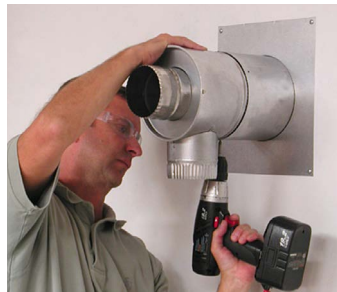
5. Assemble the tee and attach it using screws. Not a positive pressure location, but requires a good seal to prevent pressure imbalances.
