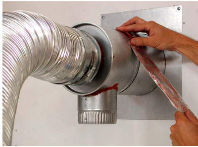
11. Seal or tape the joints from the termination to the tee assembly.
