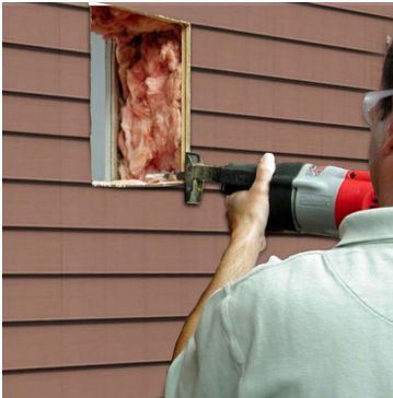
1. Select the terminal location and cut a hole through it. (See No. 4).
