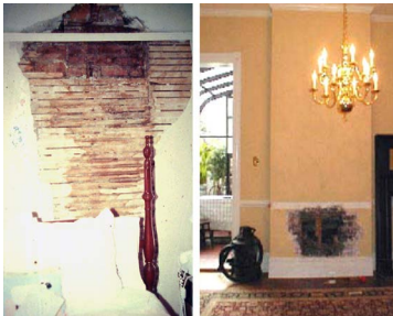
Fig. 26: Moisture or stains on interior walls near chimney
