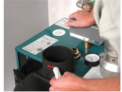
12. Apply a bead of sealant to the appliance collar.
