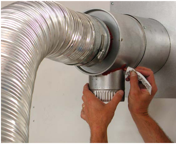
10. Apply sealant to the cover pan around the inner pipe, joints and tee assembly.
