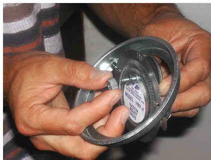
21. Install VRV close to the air inlet of the burner and adjust for proper flow.
