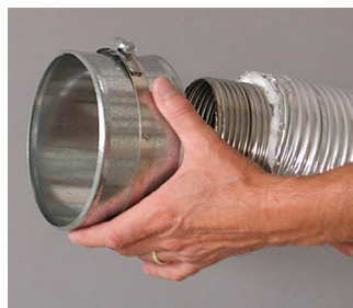
8. Place the cover sleeve onto the flue pipe.
