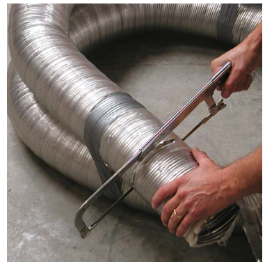
6. Cut the listed insulated pipe to the appropriate length.
