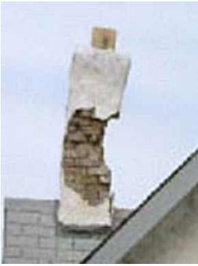
Fig. 21: Leaning chimney
