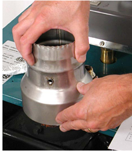
14. With a twisting motion, assemble the adapter to the appliance collar.
