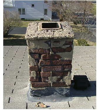
Fig/ 23: Loose bricks and/or mortar
