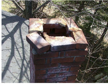
Fig. 22: Chimney crown damage
