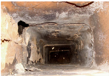
Fig. 29: Misaligned terra-cotta tiles at the joints
