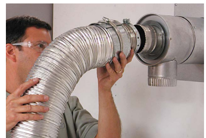
9. Attach the pipe onto the tee.
