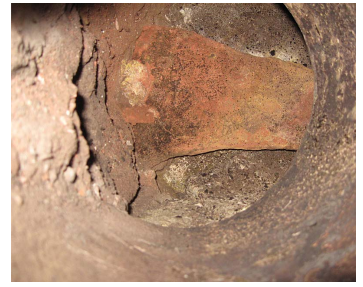
Fig. 28: Debris in the clean-out
