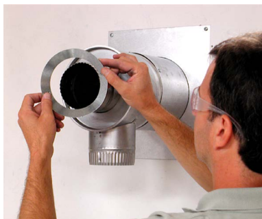
7. Place the collar on the back of the tee.
