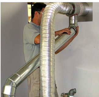
20. Install elbow into bottom of tee and run intake air pipe to burner location.
