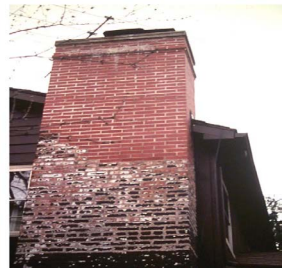
Fig. 25: Moisture on exterior walls of chimney
