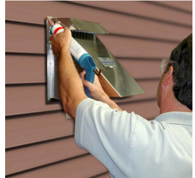
3. Mount the vent terminal through the wall from the outside, fasten and seal the edges of the base plate with high temperature silicone sealant.
