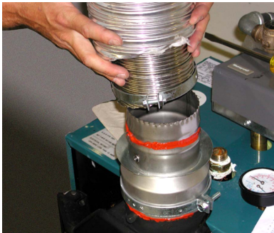
17. Attach flue pipe to adapter.
