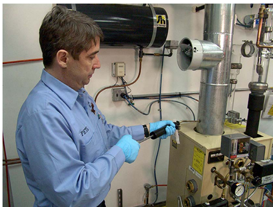
Figure 4: Technician performs a smoke test with combustion analysis results below.
