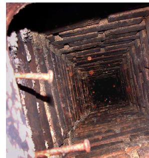
Fig. 30: No liner installed
