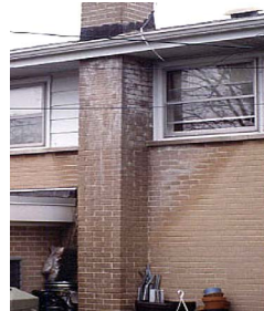
Fig. 25: Moisture on exterior walls of chimney
