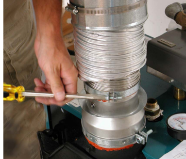
18. Adjust clamp until both halves are 1/8" apart.
