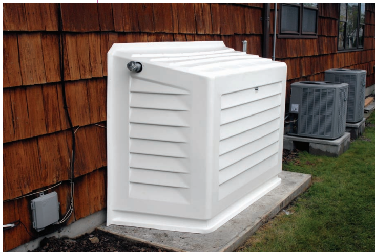
Figure 2-4: Tank shed covering an outdoor, above ground tank
