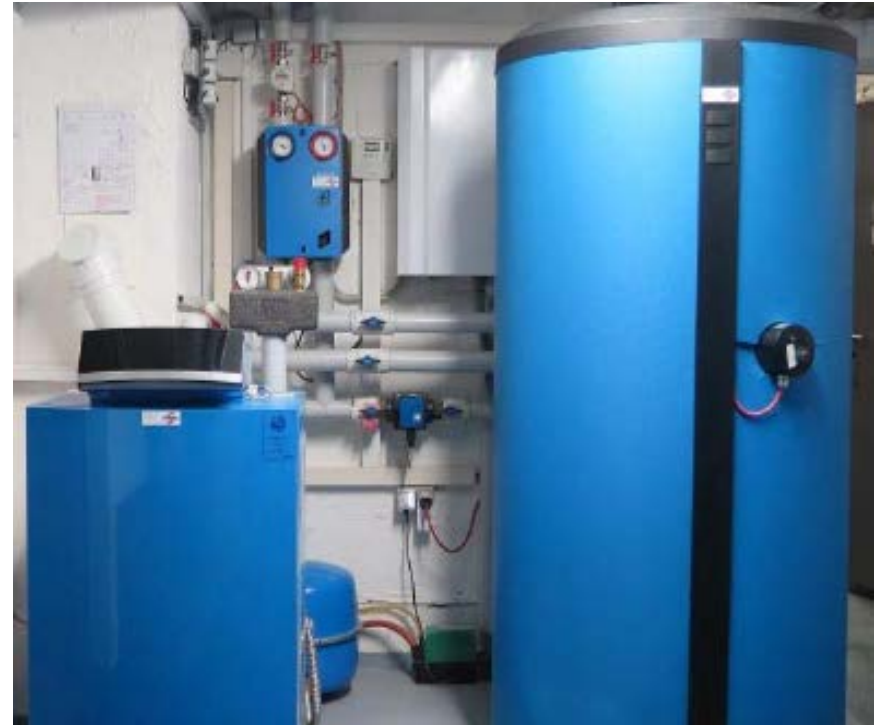
Test house in Berlin
