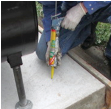
Fig. 4. Adding adhesive to the drilled hole
