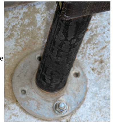
Fig. 5. Design A1 foot flange with bolt
