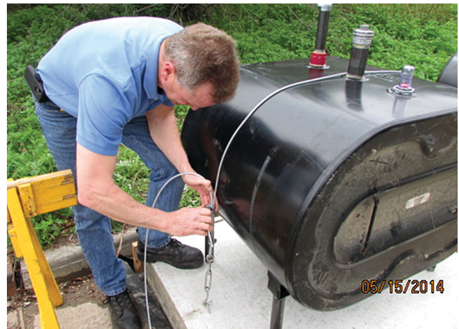
Fig. 13. Installer performing wire rope tie-down.
