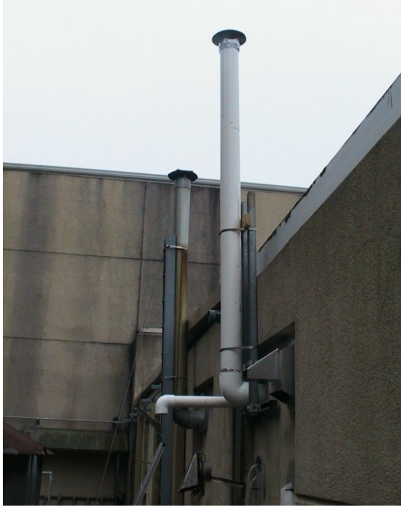
Figure 6 Photo of vertical plastic stack
